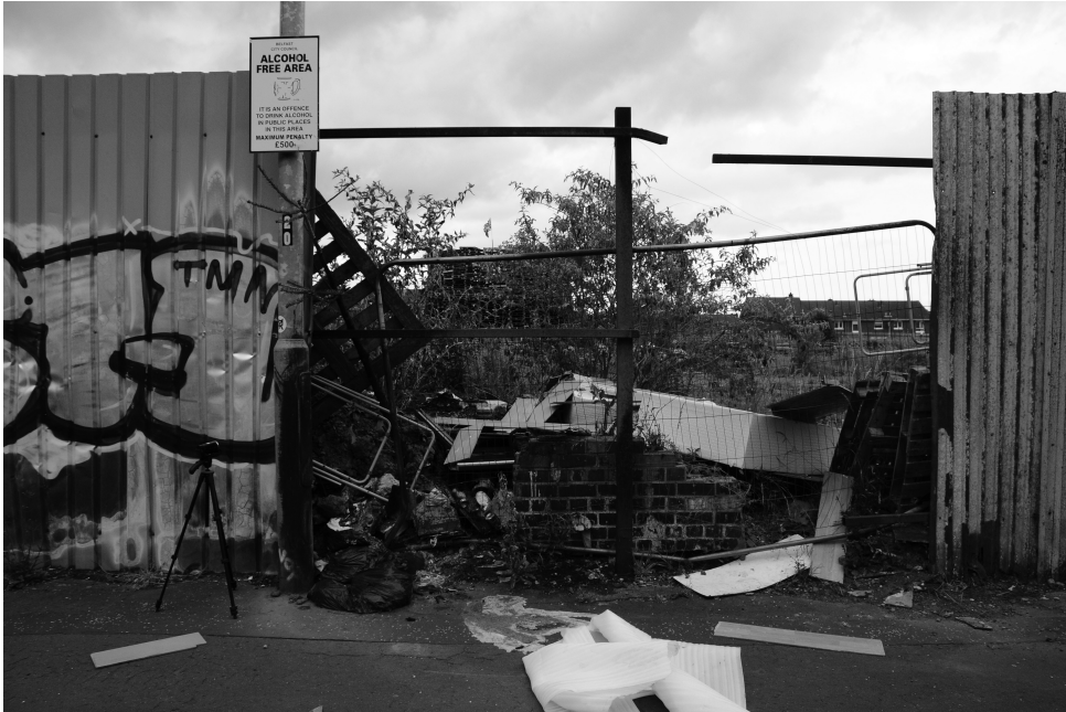
Figure 13.5 The current condition of dereliction adjacent to the Falls-Shankill 'peace line' at Cupar Way, Belfast. Photograph by James O'Leary (2020).
