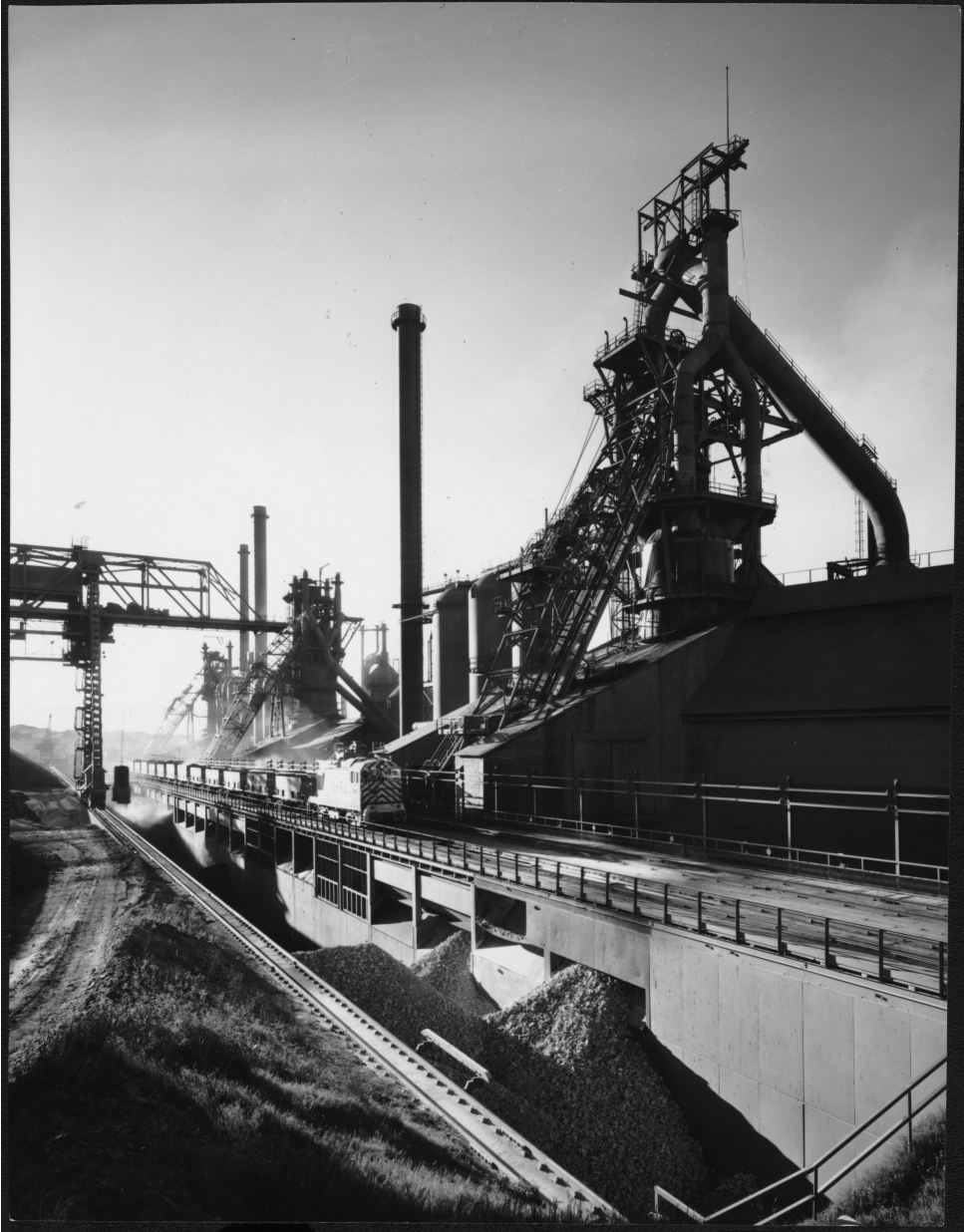
Figure 15.4 Port Kembla BHP Steelworks showing the blast furnaces with locomotive and train of hopper wagons. Mark Strizic, 1959. Source: National Library of Australia, P861/5485; © The Estate of Mark Strizic.
