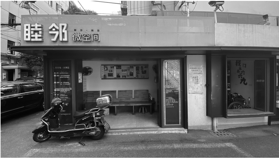
Figure 10.4 A street-facing open community space named as “for neighborliness micro-space” (or mulin wei kongjian , in Chinese). The motorbike partially blocked the entrance on the day when the picture was taken. But the space was intended as an open and inviting space for residents. Its interior space is furnished with wooden chairs and decorated with pictures relating to the stories about the community on the wall facing the entrance and some decorative signs in Chinese characters saying “This is Our Lane 669” on the wall of the right side of the picture. Photograph by Xing Xing (2020).
