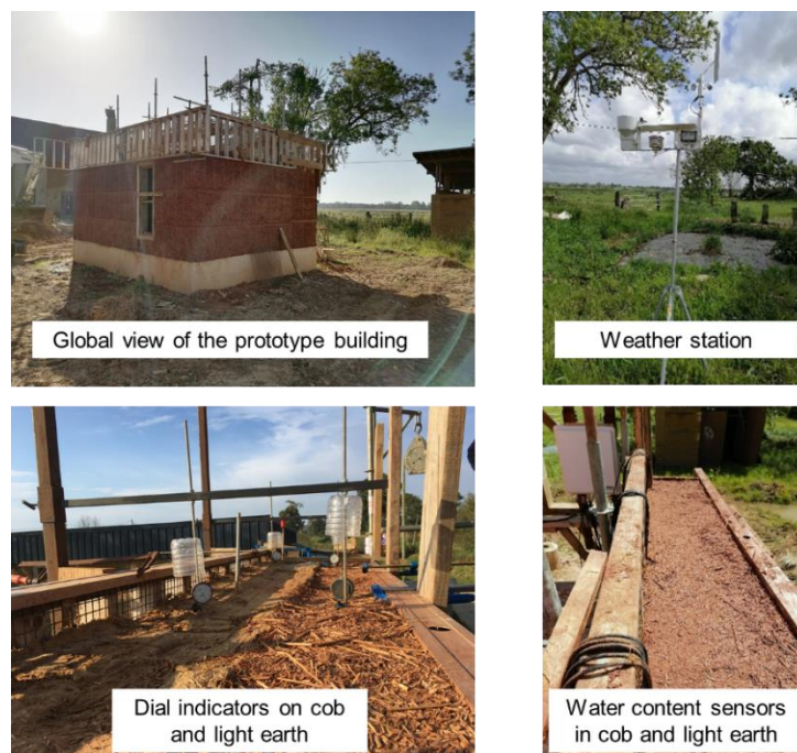
Figure 3 Global view of the prototype building, and instrumentation made on site.
