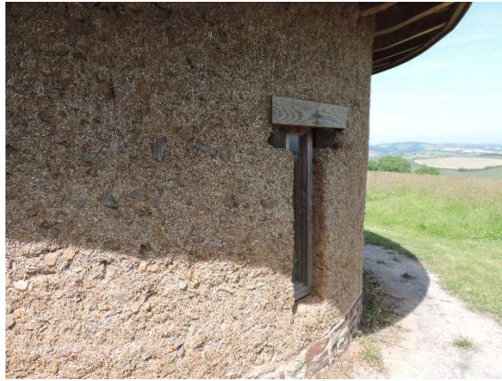
Figure 1. Exposed cob construction in Totnes, UK.
