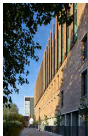
Figure 7: Exterior of AGB showing courtyard.
