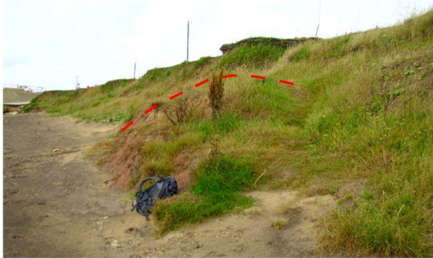
Figure 3.5 Shallow single rotational landslide (1) at Yaverland. 40L back pack for scale.
