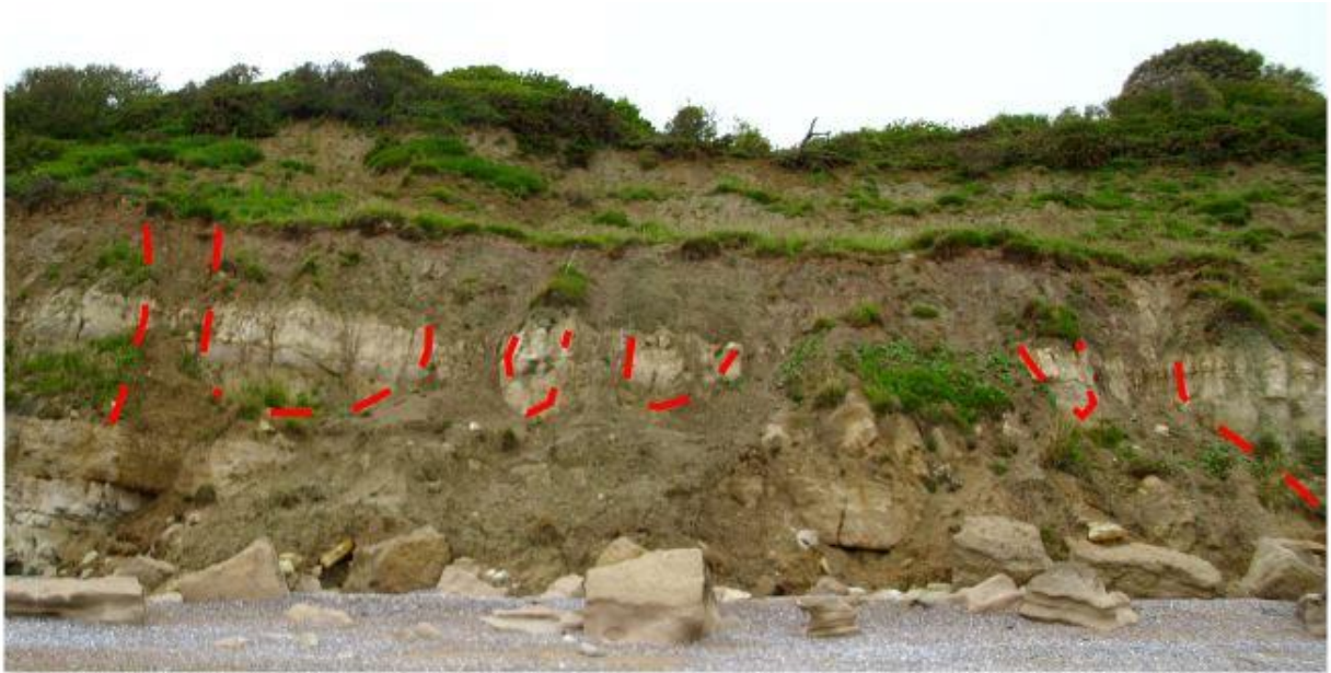
Figure 3.3 Complex landslide with main type of movement (25) being flow type (Whitecliff Bay).
