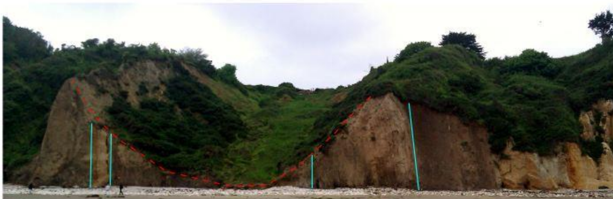
Figure 4.4 Complex landslide (9, Figure 3.12) showing the relationship between bedding surfaces and the extent of the landslide.
