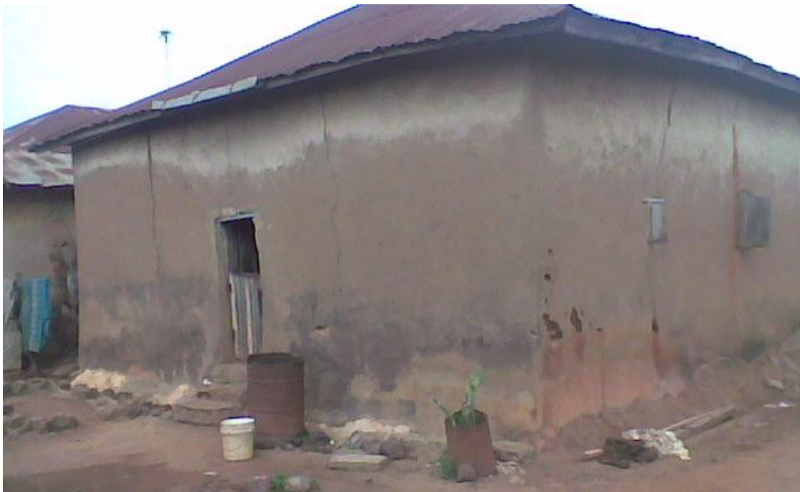
Figure 5.28: A cob building with cementitious render in Offa
