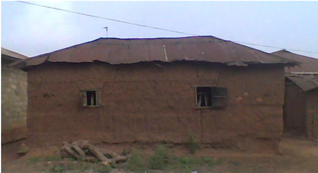
Figure 5.26: One of the cob building surveyed in Offa
