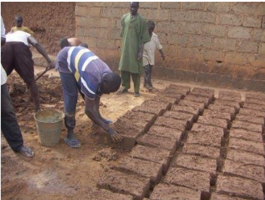
Figure 5.16: Demoulding of adobe block
