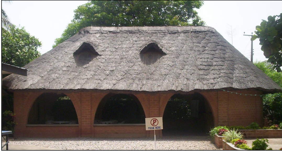
Figure 3.3: A sit-out designed and constructed by the author in 2000 in Kaduna using CEB walls and thatch roof
