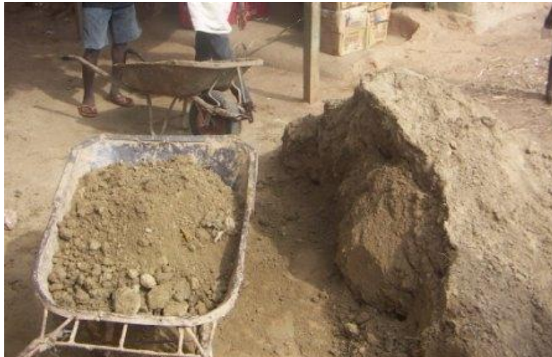
Figure 5.13: Crushed building earth ready for mixing
