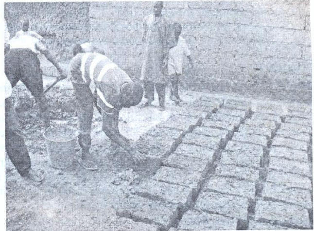
Figure 2 Adobe blocks production.
