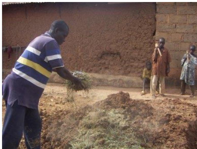
Figure 5.14: Straw is being added to wet soil mix
