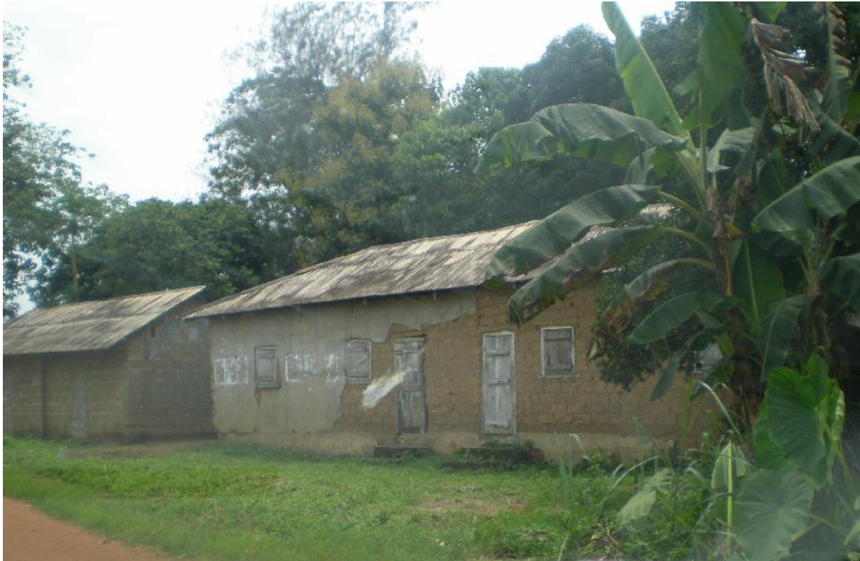
Figure 4.8: Adobe building in Ogoja, Cross River State, south east Nigeria. This is an evidence of the popularity of this technical in the southern region ©Nuhu (2006)
